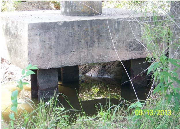
Figure 6. Pile Section Loss on a Texas Bridge with Steel Piles Under a Footing
