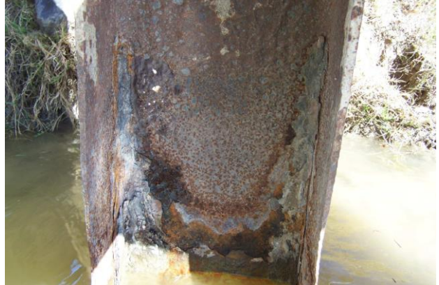
Figure 5. Pile Section Loss on a Texas Bridge with Steel Trestle Piles
