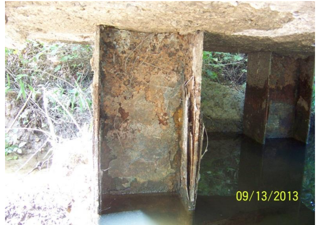
Figure 6. Pile Section Loss on a Texas Bridge with Steel Piles Under a Footing
