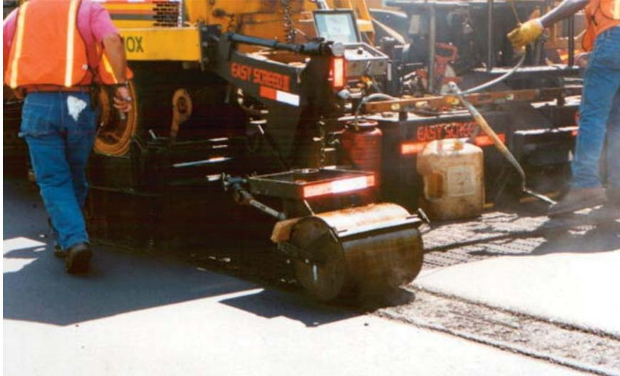
Figure 2. Compaction of a notched wedge longitudinal joint with static steel wheel roller.
