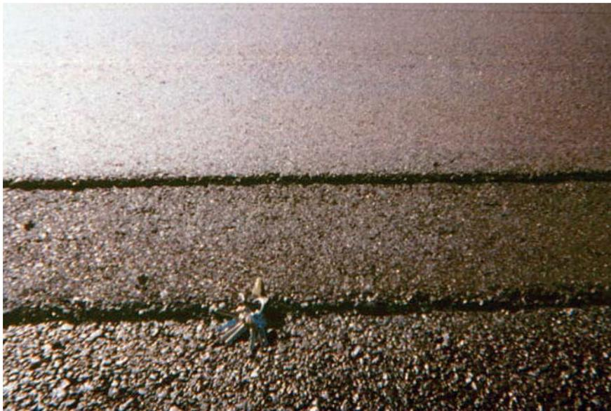
Figure 3. Notched wedge longitudinal joint after compaction.
