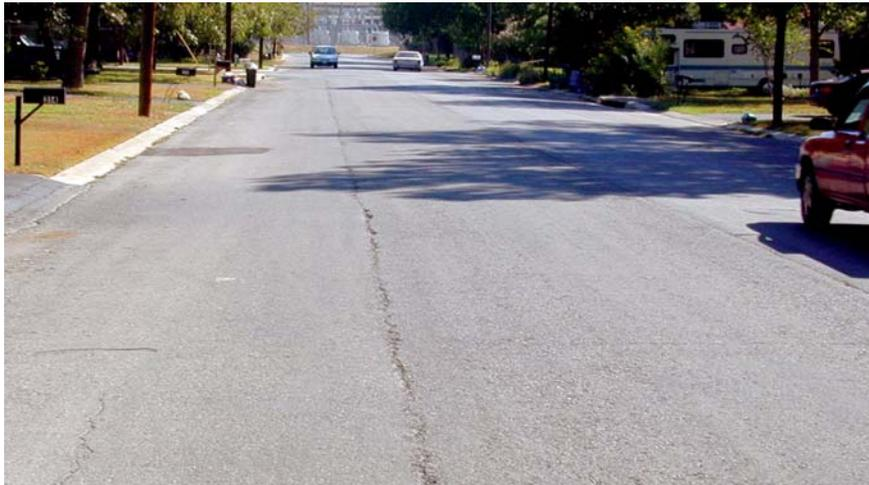
Figure 1. Poorly constructed longitudinal joint.
