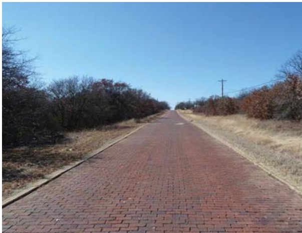
NRHP-eligible Bankhead Highway segment, Eastland Co
