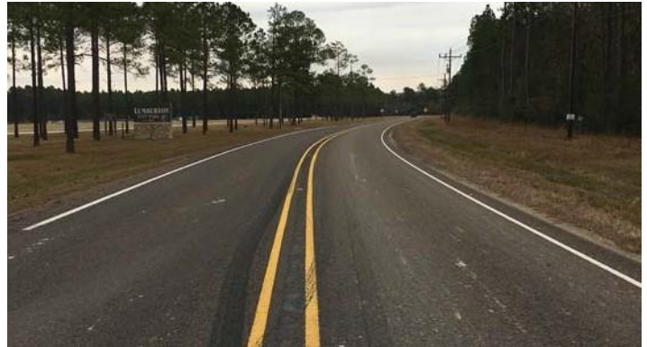
An example of a minor widening that does not affect integrity, FM 421, Hardin Co
