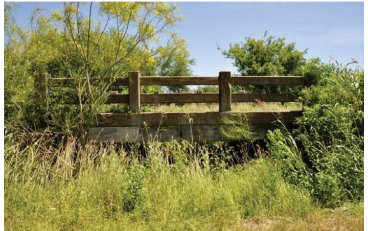
Photo of project bridge, provided by district through PCR process.
