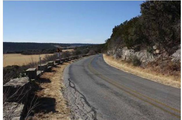
An example of an NRHP-listed Depression-Era Rd, SH 16, Palo Pinto Co
