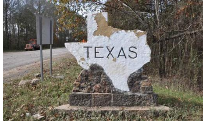
An example of an individually NRHP-eligible state line marker. The roadway itself is not NRHP-eligible, due to changes caused by widening and other loss of historic integrity.
