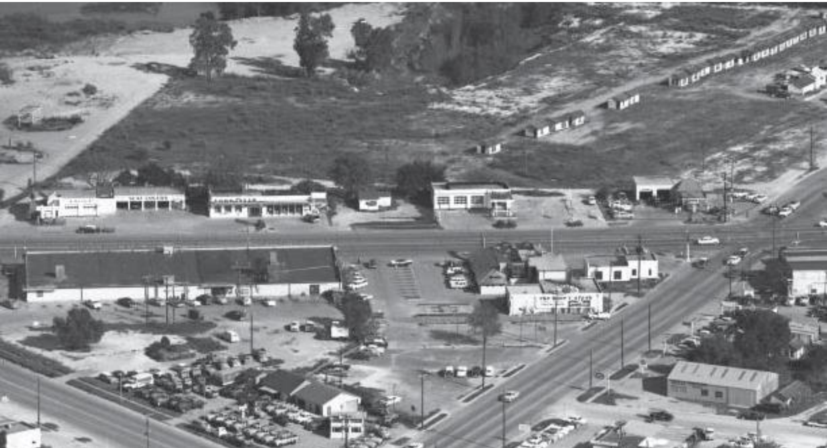
Intersection of Barton Springs Road, Riverside Dr., and South Congress Ave (Meridian Highway), view east, c. 1950
