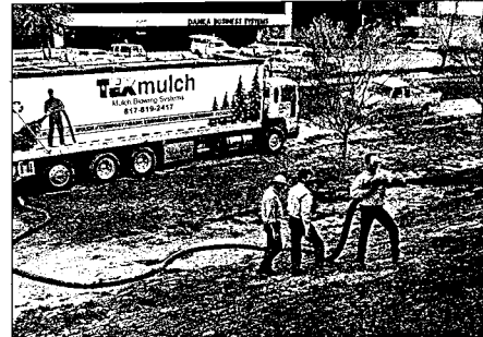
Demonstration of Erosion Control Compost application in Odessa on an overpass along Hwy 80. A mixture of compost, cotton burs and wood chips was blown-on to a depth of 1 inch by TEX-mulch specialists Joe Hardac and Greg Hatch.
