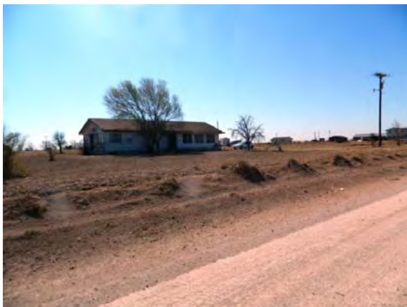
Figure F-4: Ca. 1950s side-gabled residence.
