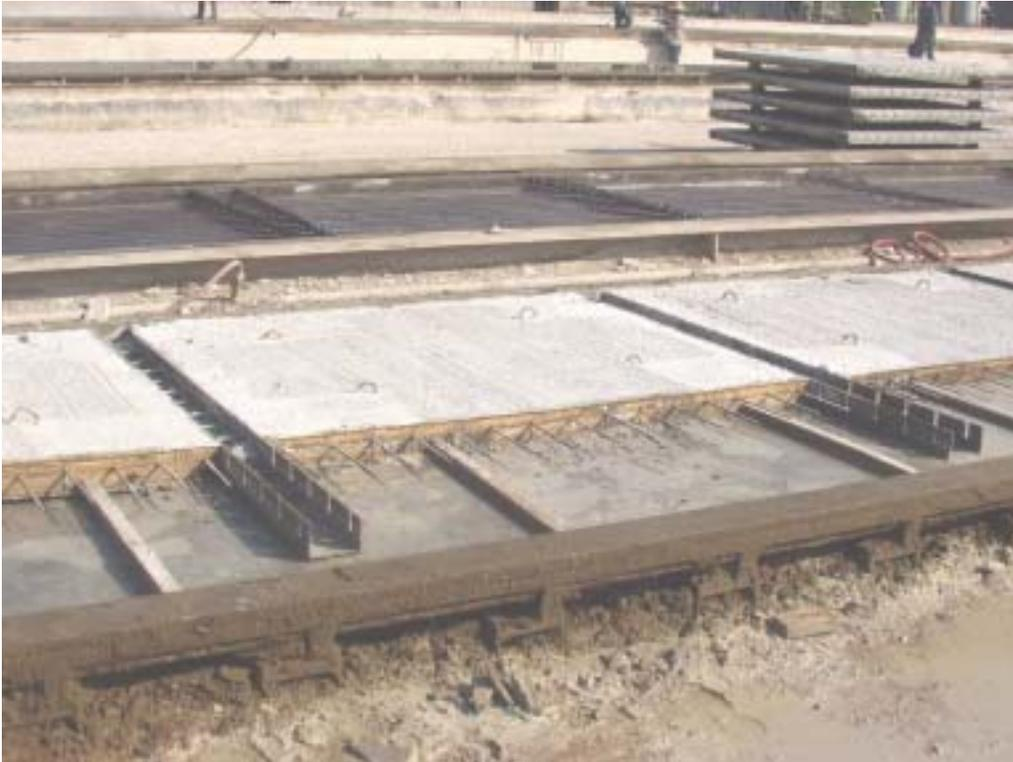
Fig. 5 Forming of End Panel Showing Gap in Forms and #3 Reinforcing Steel
