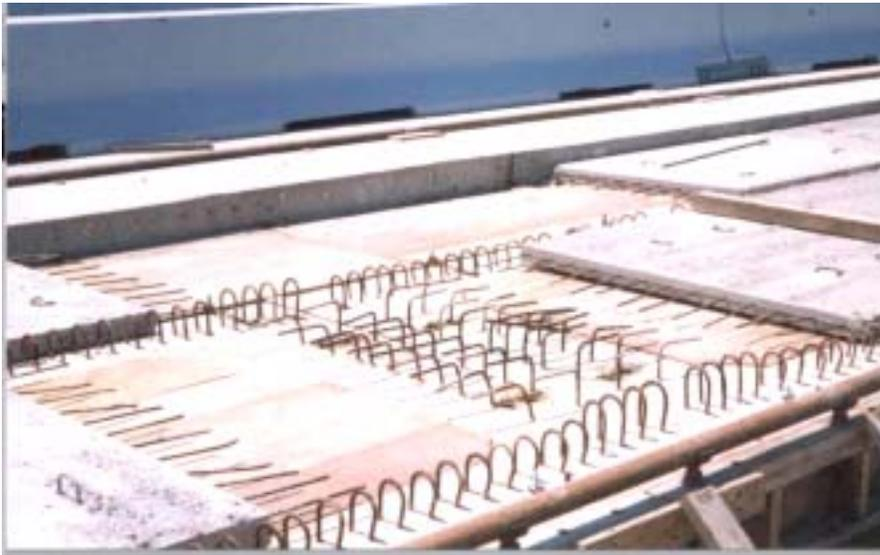
Fig. 2 Skewed Panels on 45° Skew. Note Extension of Reinforcing Steel From Panels
