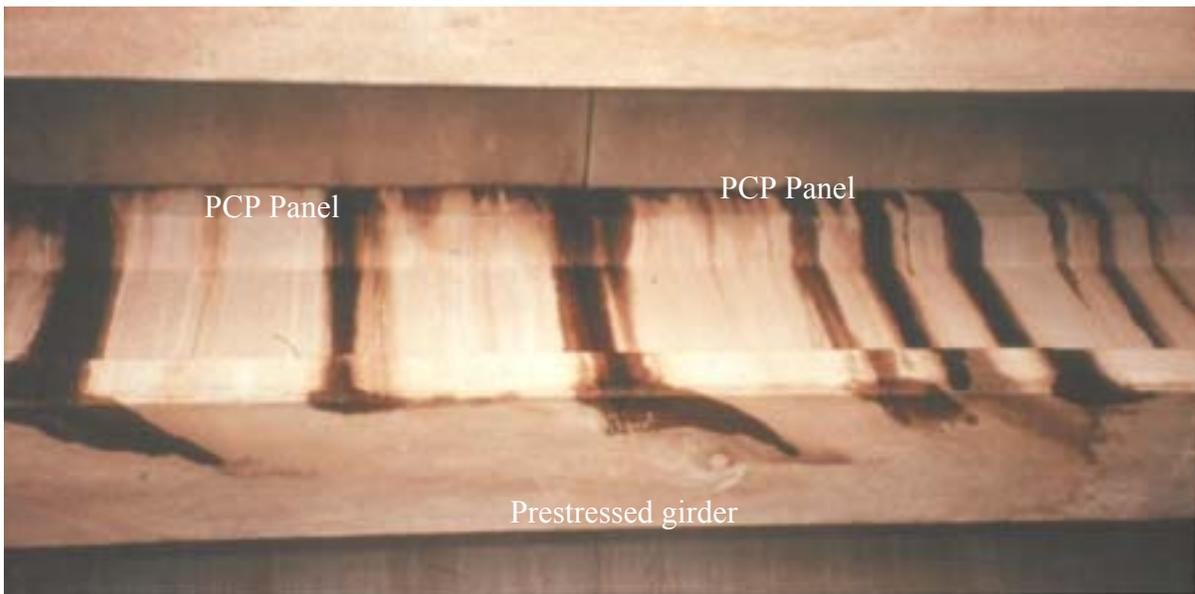
Fig. 10 Water Penetration at Crack from Fig's. 8 and 9
