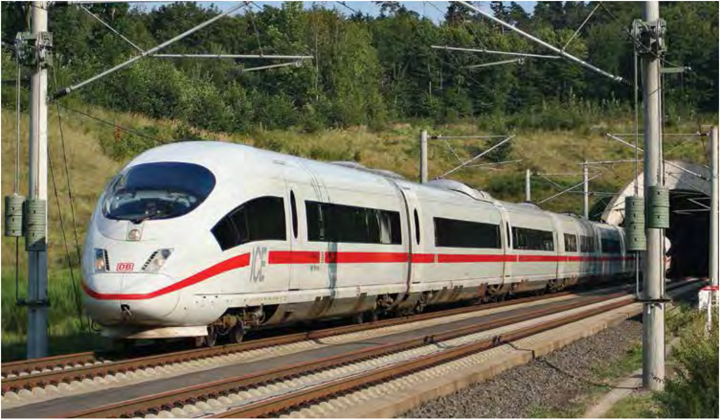
An ICE 3 high speed train on the Frankfurt-Cologne high-speed rail line, near the Oberhaider Wald Tunnel
