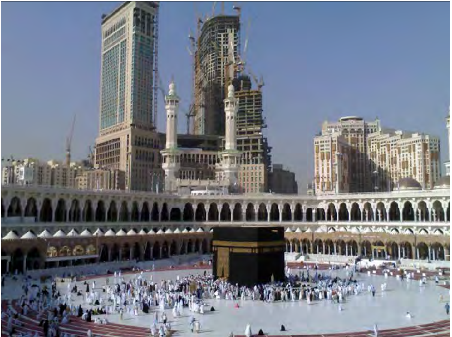
Makkah (Mecca), Saudi Arabia. A high speed inter-city rail line (Haramain High Speed Rail Project also known as the “Western Railway”), is under construction in Saudi Arabia. It will link along 444 kilometres (276 mi), the Muslim holy cities of Medina and Mecca
