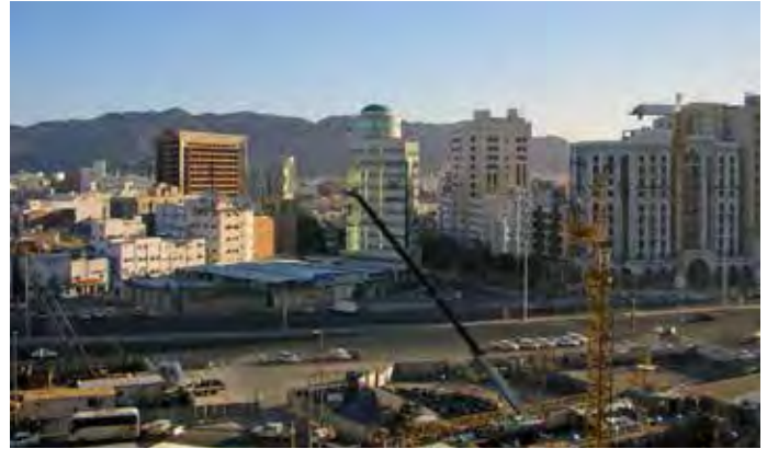
Medina, Saudi Arabia. The Haramain High Speed Rail project will link the two cities of Medina and Mecca.
