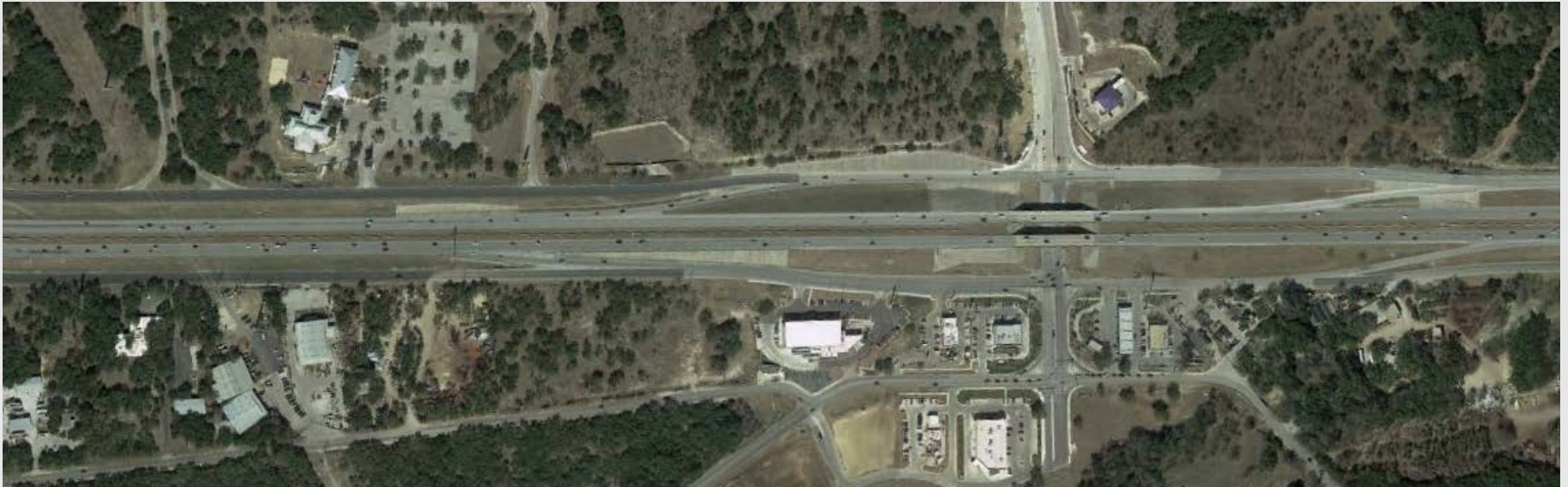
Visual of Typical Expressway
