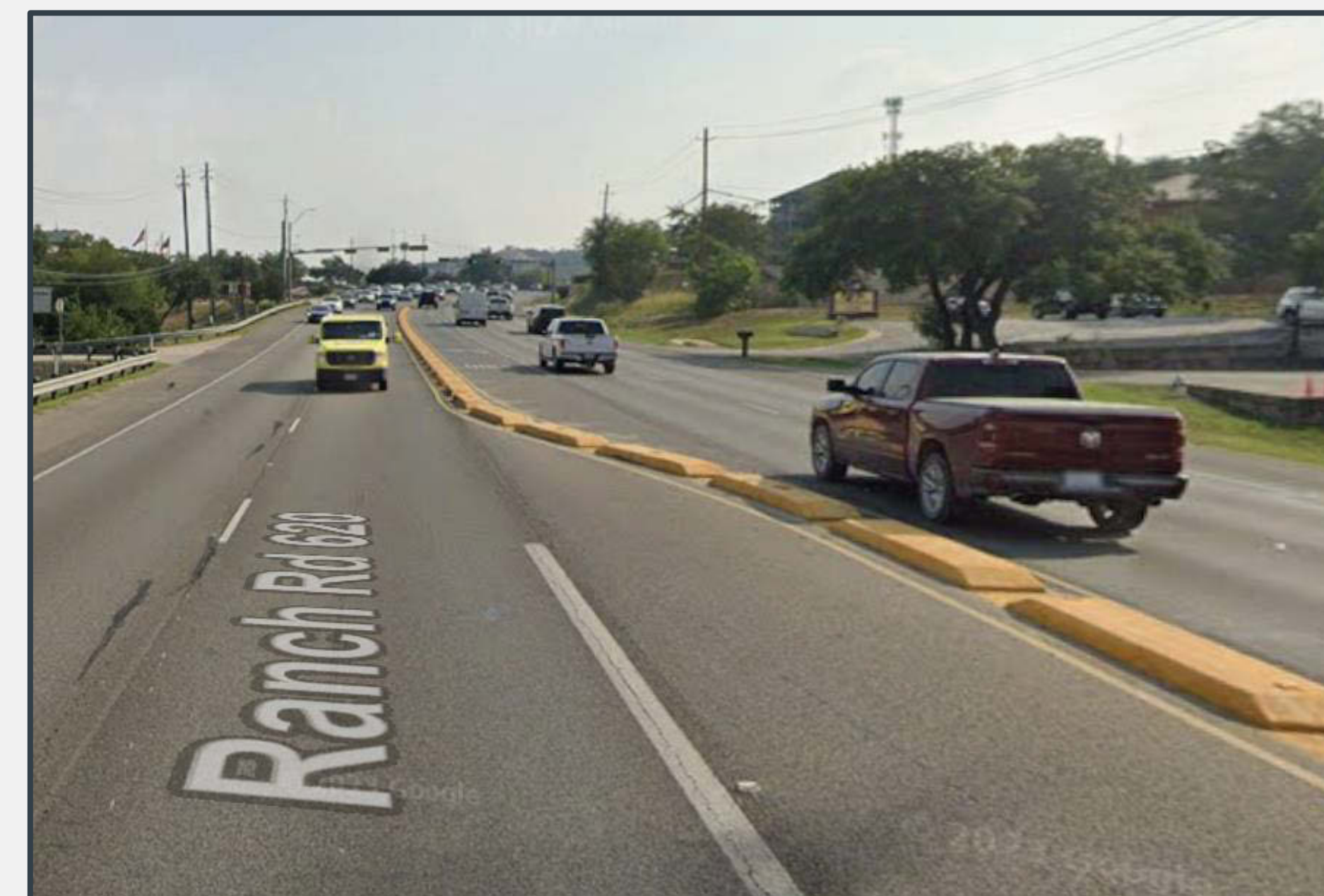
Median at Two Traffic Lights
