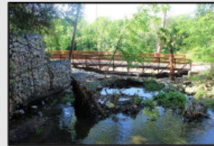
Brushy Creek Trail bridge south of culvert
