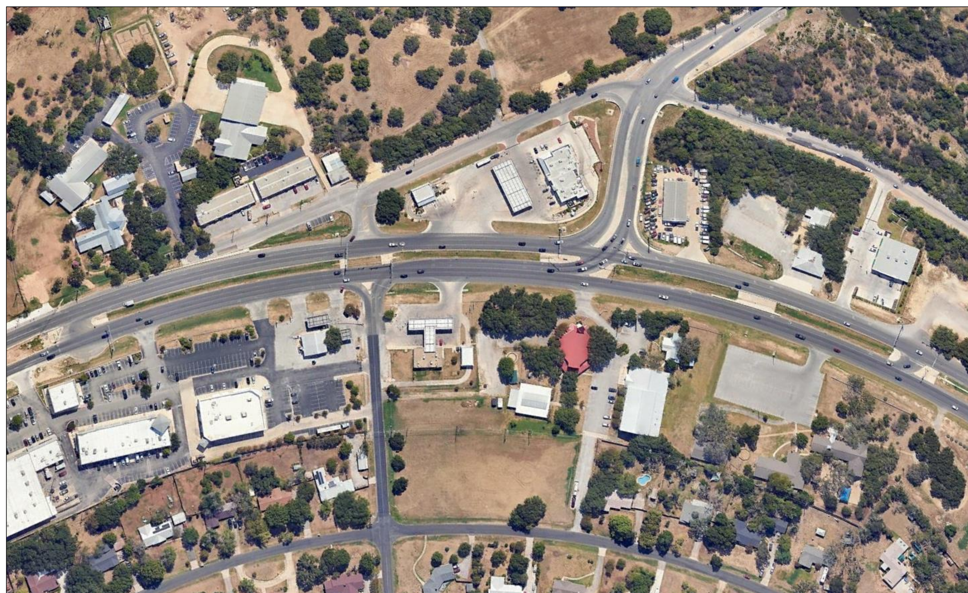
R-CUT in San Antonio at SH 16 (Bandera Road) and FM 1560
