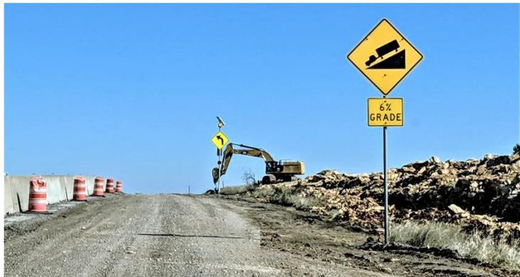
*Barriers separate the area where traffic has been shifted at the top of Ranger Hill on the south (eastbound) side of I-20. Once the project is complete, the new I-20 incline will be about half as steep as its current 6 percent grade.*
