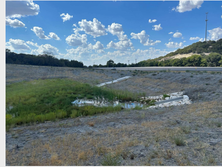
Existing US 190 Improvements project area
