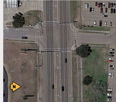
Aerial image of FM 624 at River E Dr with center turn lane
