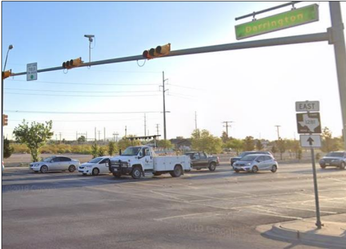
Figure F.3: Video Detection Camera Installed on the Traffic Signal Mast Arm at Horizon Boulevard at Darrington Road
