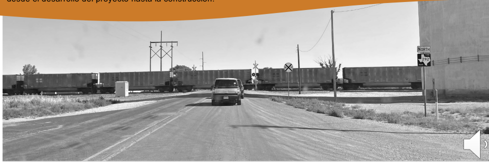
Farwell Railroad Bridge Project
