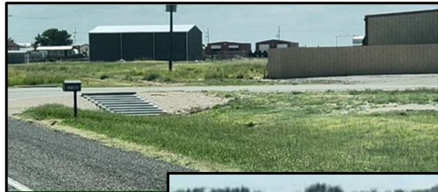
At Bailey Boiler Works, south of Woodrow
