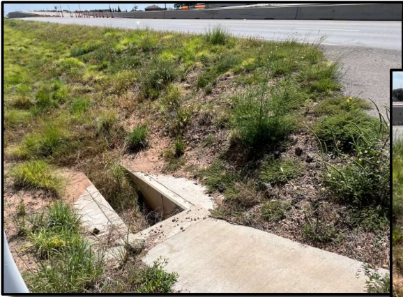
Steep, south-facing culvert at my drive
