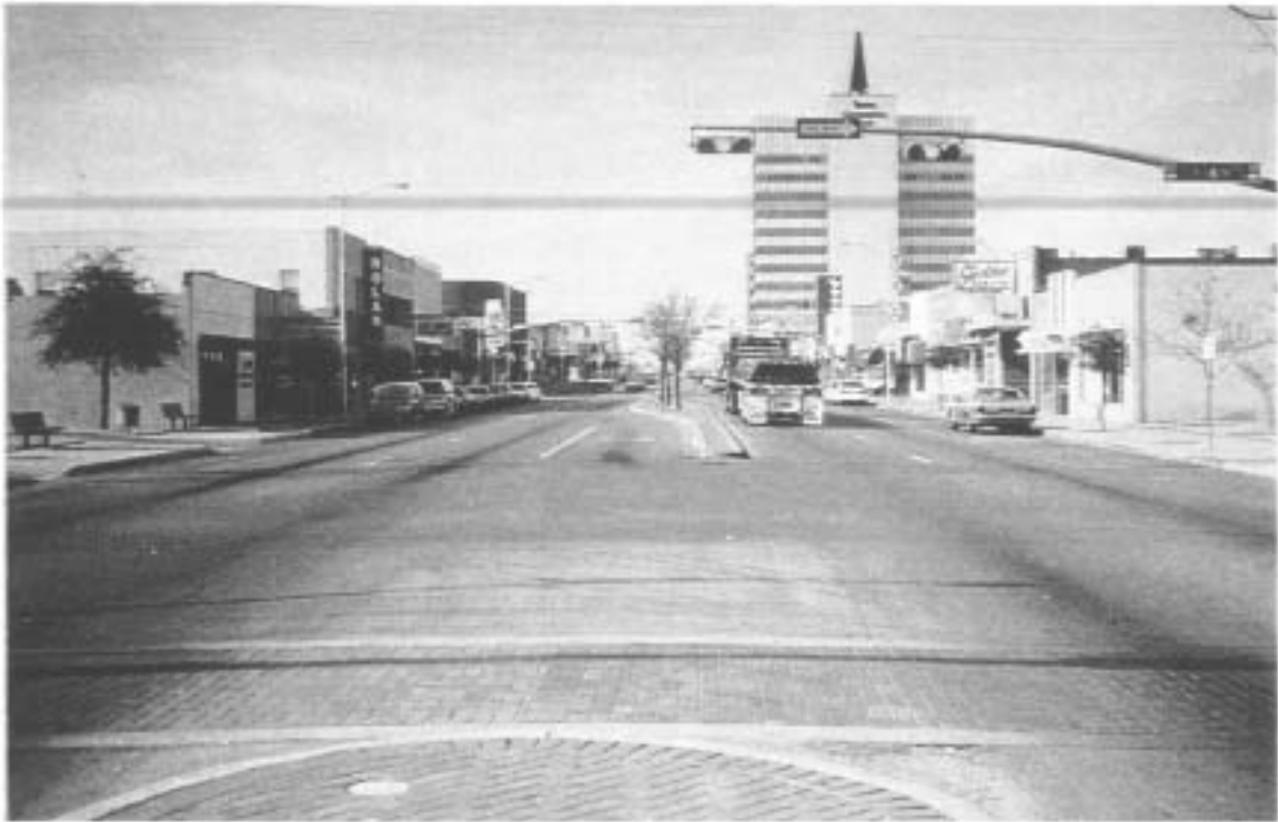
Figure 2-33. Northbound Grant Avenue at 4 th Street.
