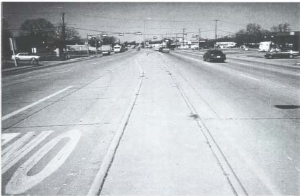
Figure 2-23. Westbound University Drive near Church Street.
