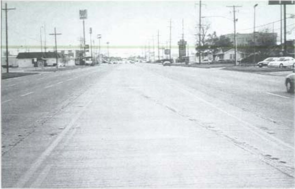
Figure 2-19. Southbound Twin Cities Highway North of Texas 73.
