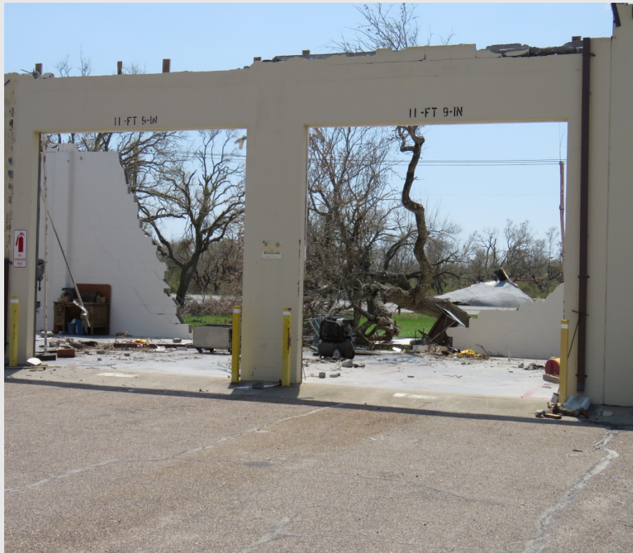
TxDOT's Rockport maintenance facilities
