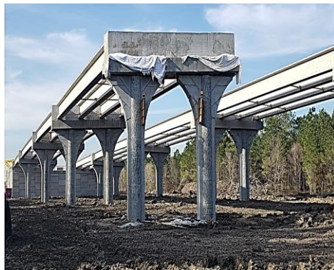
Figure A.3: Bridge 1 Beam Installation in Segment H2
