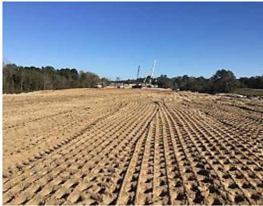
Figure A.2: Embankment work in Segment H1C
