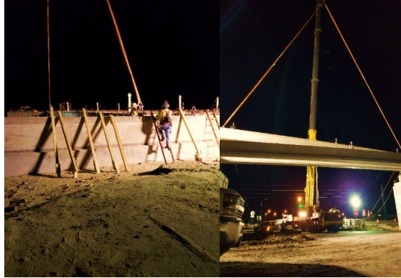
Figure A.7: Beam Set for Bridge 16 in Segment I2A1
