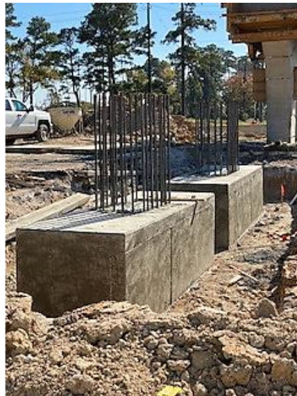
Figure A.9: Bridge 26 Wyoming Drill Shafts in Segment I2B2
