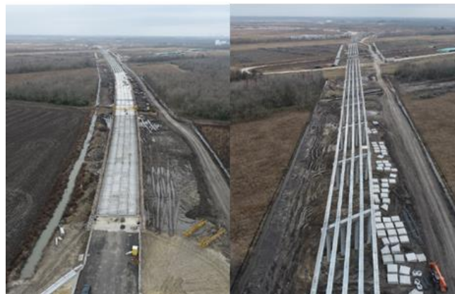
Figure A.6: Bridge 8 in Segment I1A
