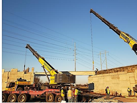
Figure A.4: Bridge 262 Beam Installation in Segment H2
