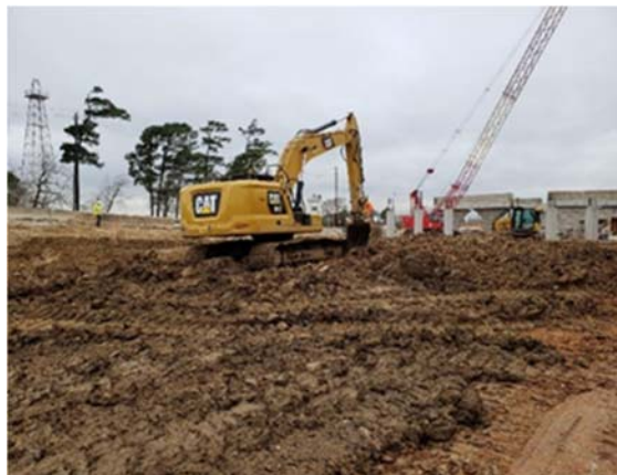
Figure A.9: Embankment at Westbound Mainlanes in Segment I2B2
