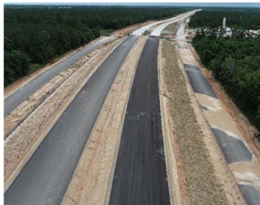
Figure A.3: Bond Breaker in Segment H1C
