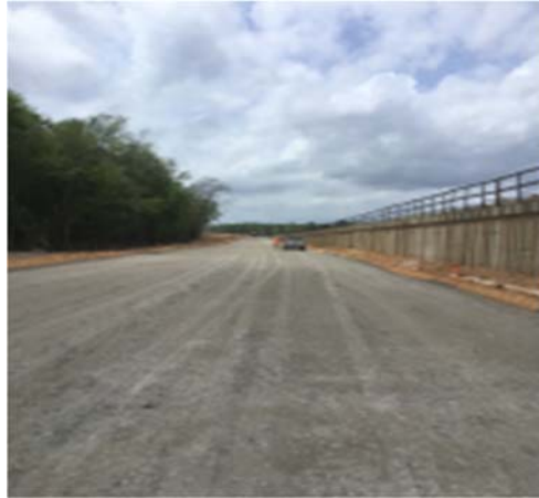
Figure A.1: Cement Treated Base Placement in Segment H1A
