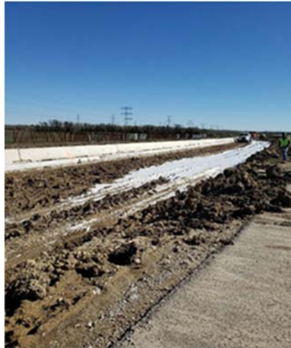
Figure A.8: Lime Placement on Ramp 10 in Segment I2B1
