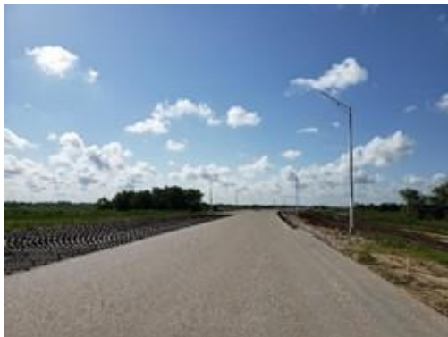
Figure A.4: FM 1960 Light Pole Installation in Segment H2
