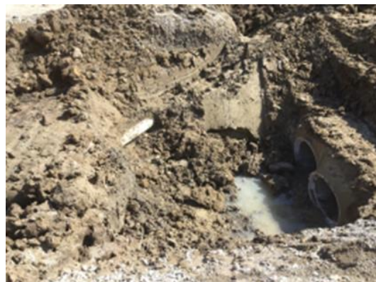
Figure A.3: Placed Pipes and Culverts in Segment H1B
