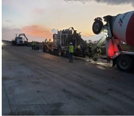
Figure A.7: Kilgore Barrier in Segment I2A1
