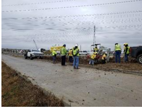
Figure A.10: Drilling for ITS Pole in Segment I2B1
