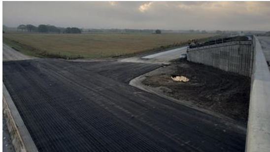
Figure A.4: Preparing FM 1960 for Concrete Pour in Segment H2
