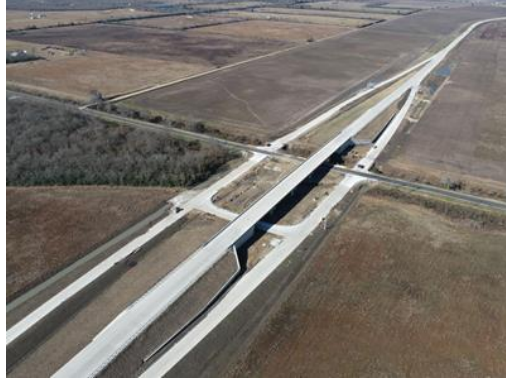
Figure A.7: Completed Pavement of Ramps 13C and 13A in Segment I1A
