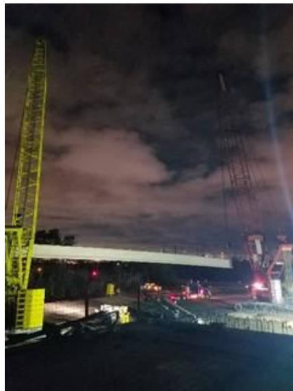
Figure A.8: Setting Beams for Bridge 10 in Segment I1A
