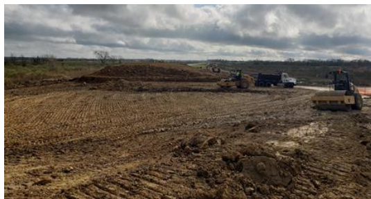
Figure A.5: Gas Line Embankment in Segment H2
