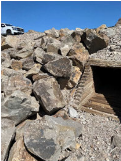
washout-prone areas refurbished
