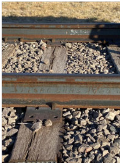
115 pound new rail relays west of Fort Stockton to enable international traffic
