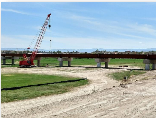
Exhibit ES - 8: Rail Bridge Reconstruction
