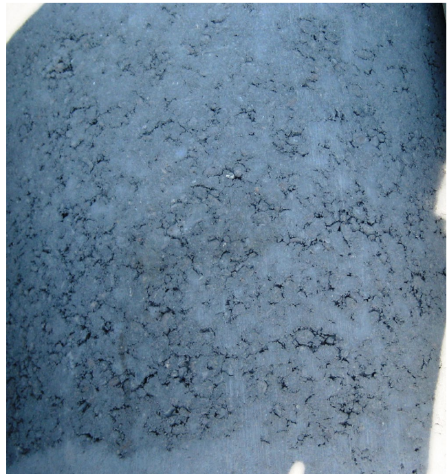
Figure 60-2—Honeycombed Concrete
