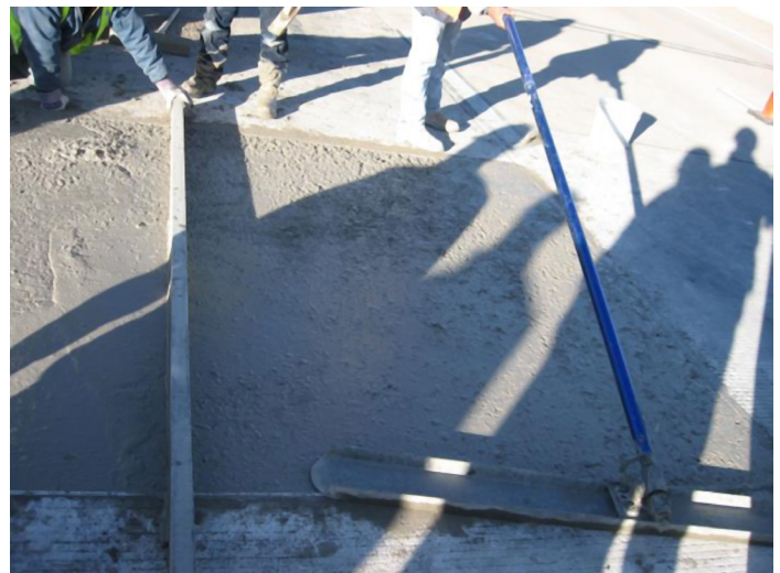
Figure 5: Finishing of CAC Concrete
