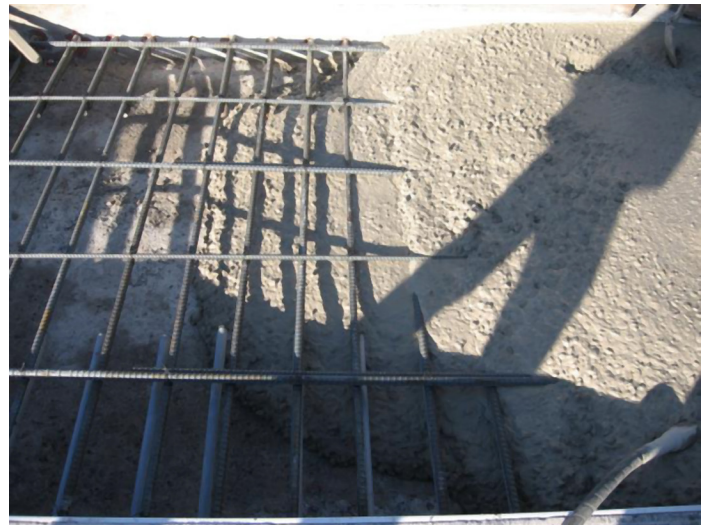
Figure 4: Pouring of CAC Concrete
