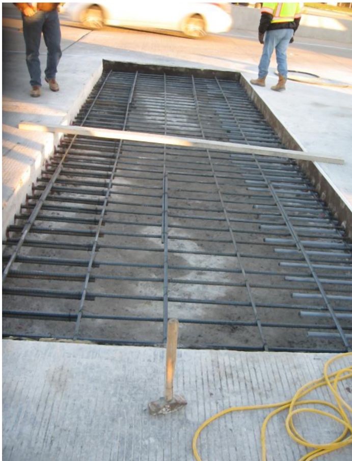
Figure 3: SH 45 Section Repaired with CAC
