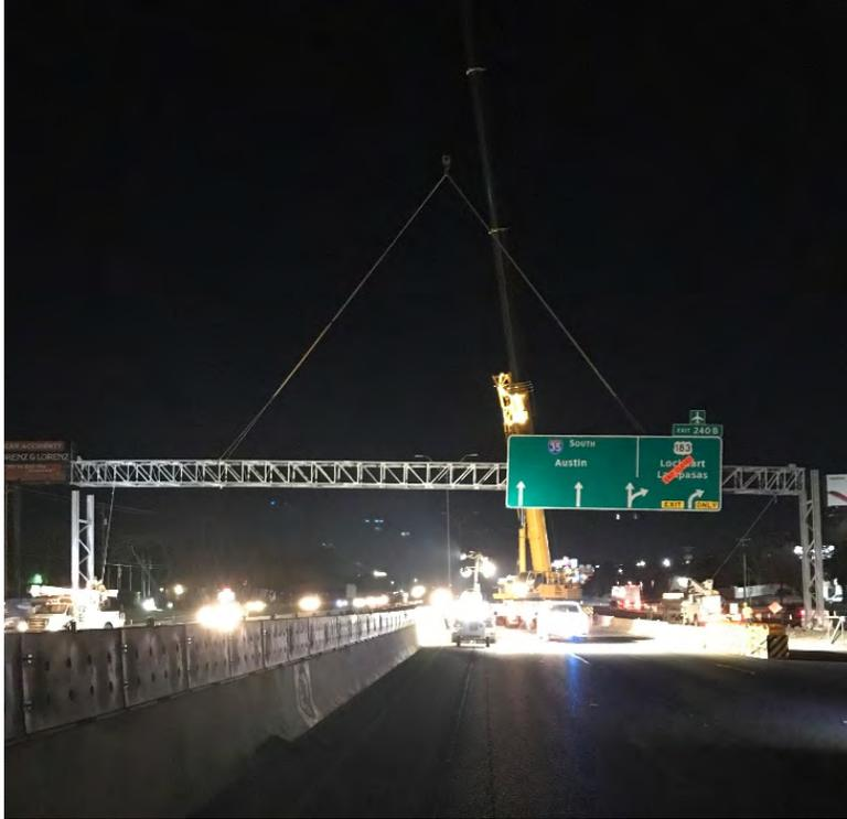
*Installation of overhead sign bridges at Rundberg Lane*
